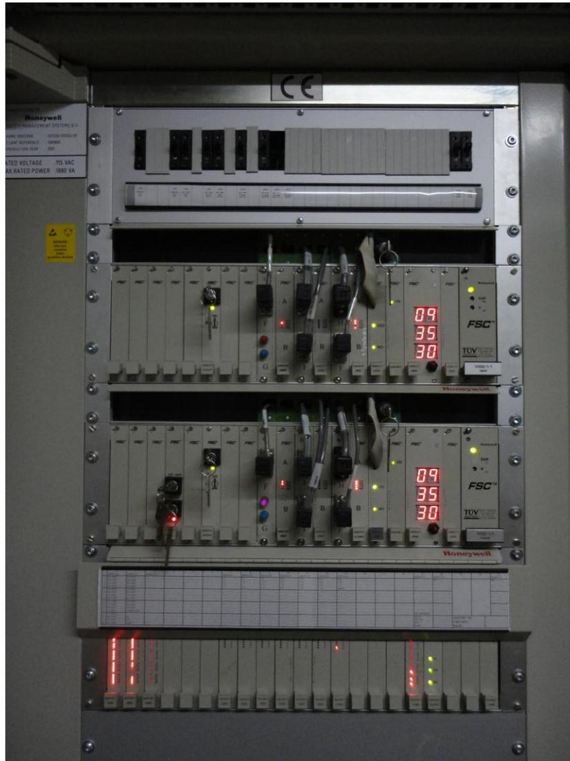
Figura 46. FSC Honeywell
