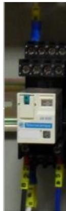
**Figura 32.** Relé universal Schneider Electric.
