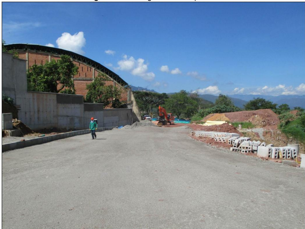
Figura 98. Base granular compactada
