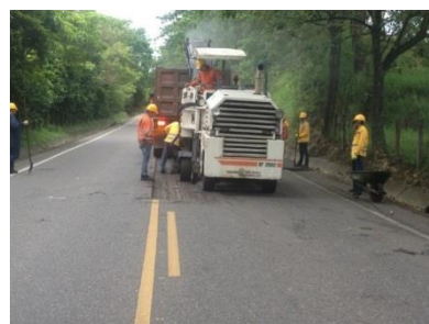
Figura No. 11: Fresado
