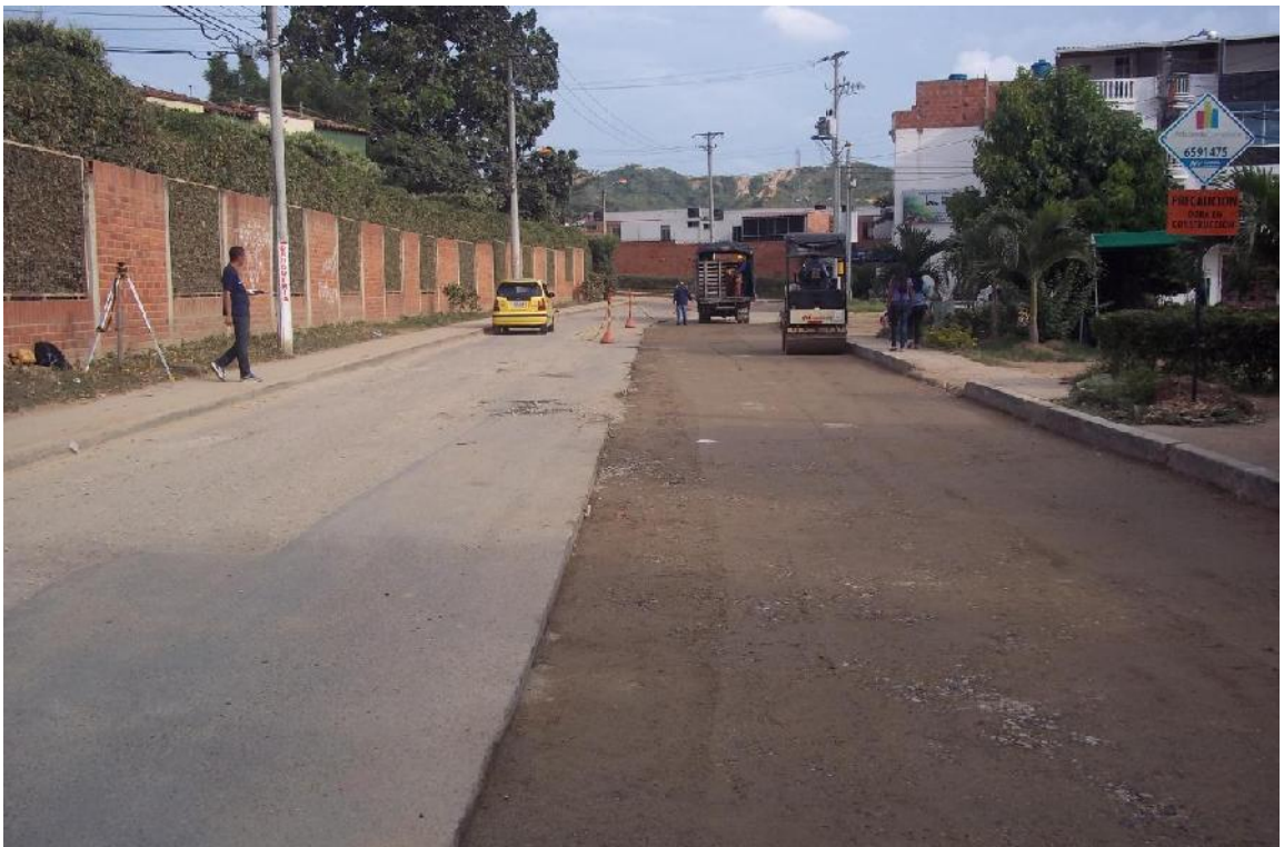
Figura 13 Base granular compactada
