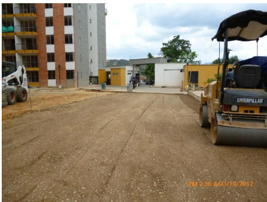
Figura 35 Base Granular compactada
