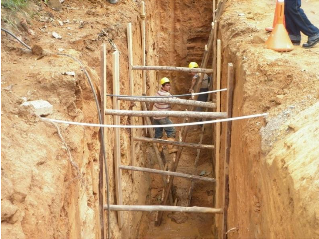
Figura 48 Entibado Pr 122-Pr 120
