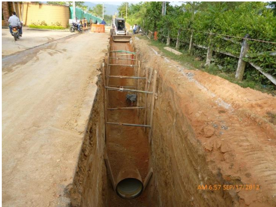
Figura 56 Relleno Pr 128-Pr 127
