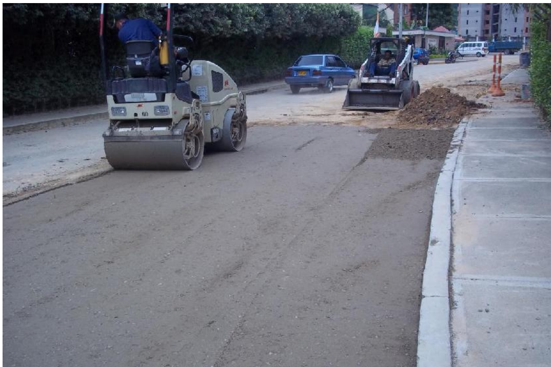
Figura 24 Base Granular Compactada
