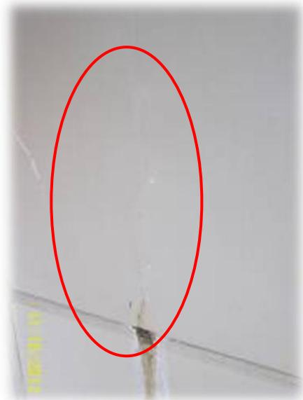
Figura 29 Fisura L/2 vertical.
