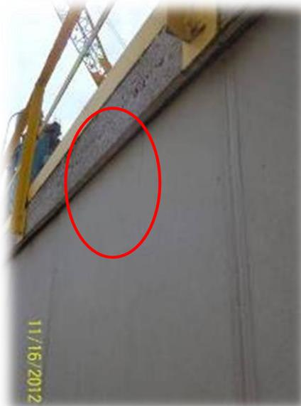
Figura 30 Fisura L/2 vertical.
