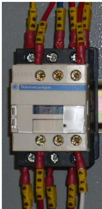
Figura 84: Contactor Tripolar LC1D18 [17]
