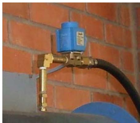
Figura 152: Válvula ON/OFF [17]
