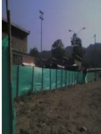
CERRAMIENTO PROVISIONAL Figura No. 6
