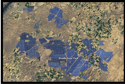
Figura 2 Bhadla Solar Park
