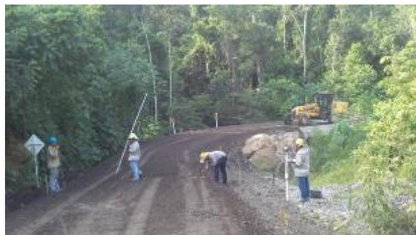
Imagen 41 Subbase Granular
