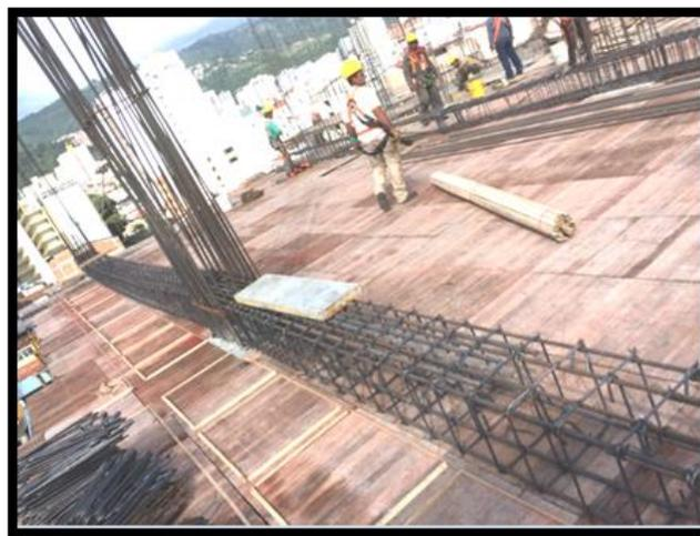
**Figura 9. Armado Viga V5 in situ**
